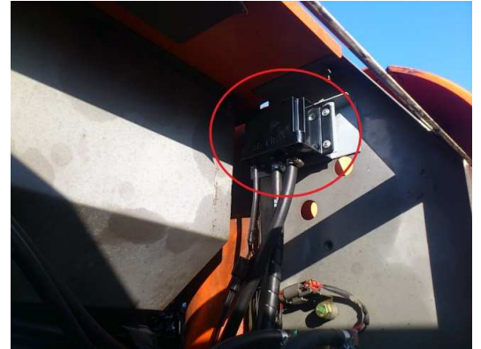
Install IKM-300 in Pump room
